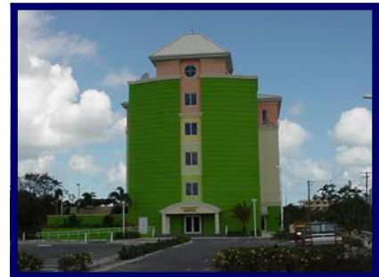
Figure 38: A CO was granted to Citrus Grove Office Project
