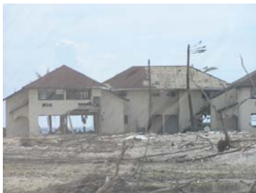
Figure 16: One of the many buildings assessed by structural inspectors.
