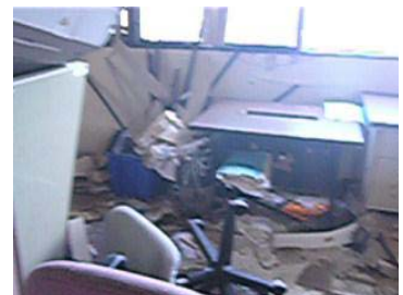
Figure 20: Planning Department offices after Ivan
