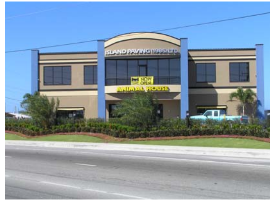
Figure 26: This mixed use of office and retail opened at the end of 2005.
