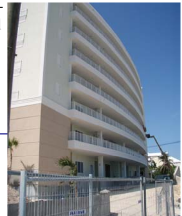
Figure 15: One of several new condo complexes on Seven Mile Beach.
