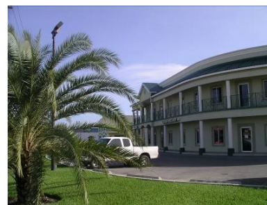
Figure 18: A new mixed-use office and retail center near Owen Roberts Airport.
