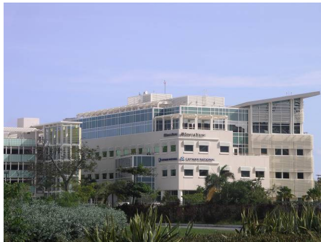
Figure 26: Construction continues at Camana Bay, a "New Urbanist" town off West Bay Road
