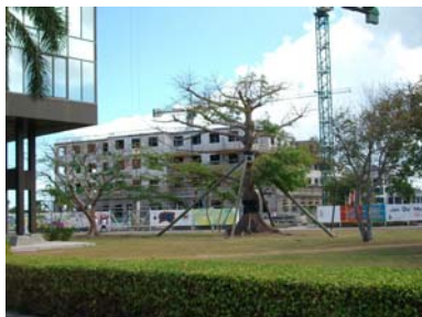
Figure 19: Government Office Accommodation Project under construction, George Town
