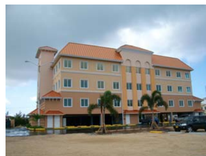
Figure 20: A new office building off West Bay Road.
