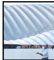
Figure 14: Building Inspector Ernesto Carter performing damage assessment post Hurricane Paloma
