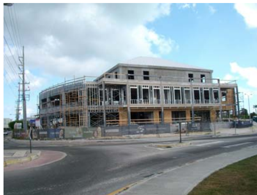
Figure 11A: Commercial building under construction at West Bay Road
