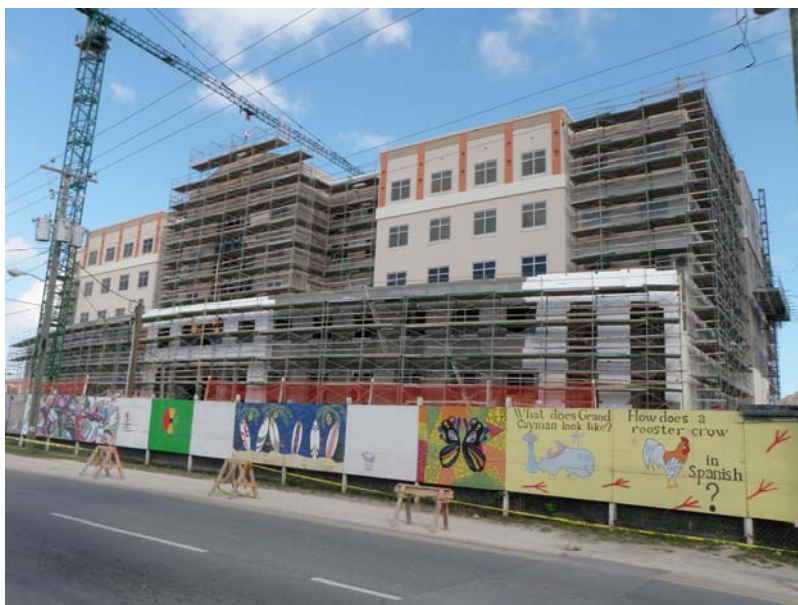
Figure 20: Government Office Accommodation Project under construction, George Town
