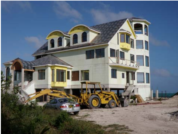
Figure 27: House under construction at South Sound Rd.
