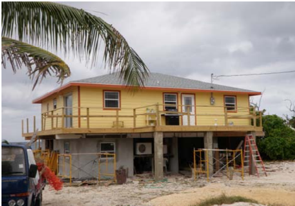
Fig. 13a: Rehabilitated Building in Cayman Brac
