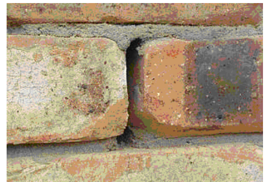
Figure 13.4 - Providing weep-holes for groundwater drainage will help the longevity of a seawall.
