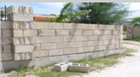
Unfinished Concrete Masonry Units
