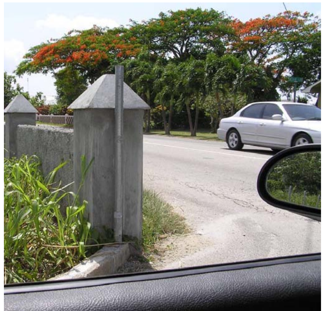
Figure 3.3.4. - An example of poor visibility due to lack of a sight triangle.
