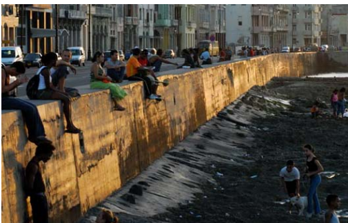
Figure 13.7(a) and (b) - Seawalls need not act as barriers to access, as seen in these examples (Vancouver, Canada and Havana, Cuba)
