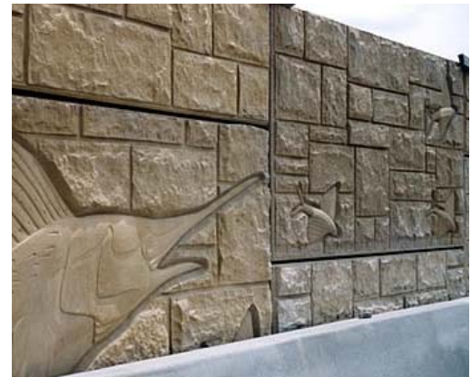
Figure 13.3 - The use of patterned concrete can help break up blank surfaces.
