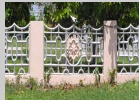
Pre-cast Concrete Panels
