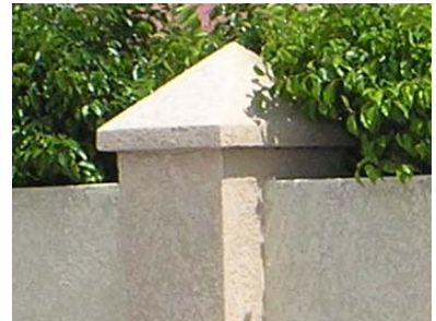
Examples of pier caps design to shed water
