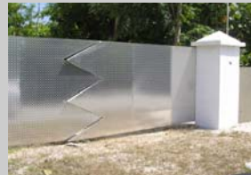
Highly Reflective Sheet Metal Panels
