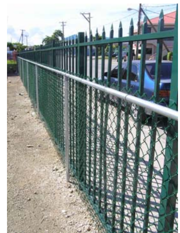
Figure 3.4.4. - An example of two redundant fences
