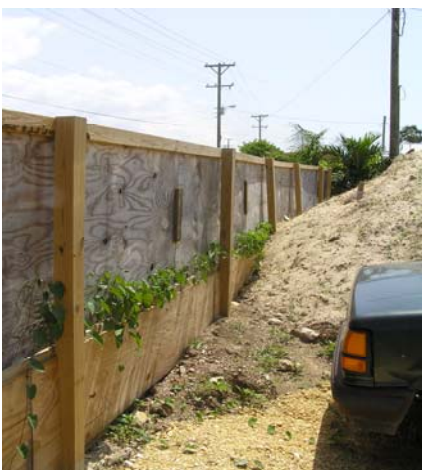
Figure 12.2.6. - Construction fencing should not be used for retaining fill.
