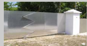
Highly Reflective Sheet Metal Panels
