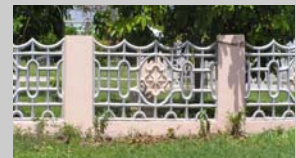
Pre-cast Concrete Panels
