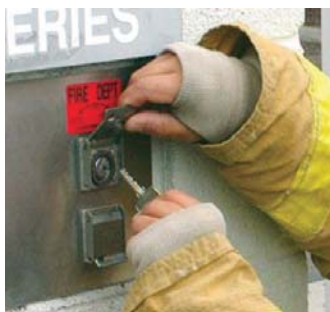
Figure 8.2.5. - Lock box containing entrance key
