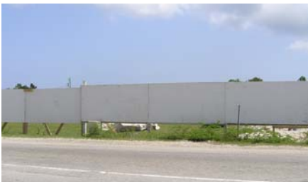
Figure 12.2.2. - Materials used in temporary construction fencing can include plywood
