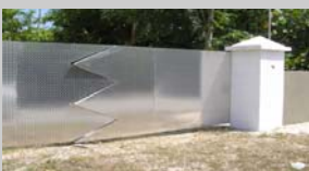
Highly Reflective Sheet Metal Panels
