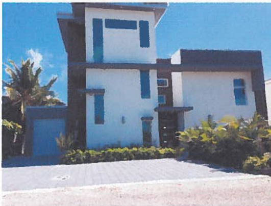
Old Prospect Rd. residence received a CO in 2013—George Town
