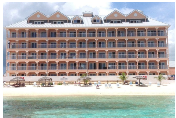
Certified Hotel/Condo Building (Londoner)—East End
