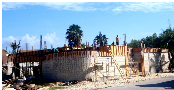
Permitted Commercial Structure (J.S. Liquors)—West Bay
