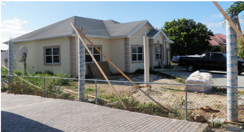
An Example of a Compliance Case (illegal structure)—Bodden Town
