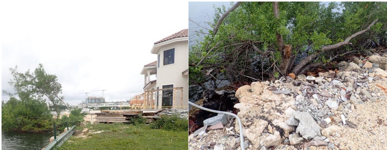
Figures 7 and 8, Loose materials and construction debris being stored on the canal side of a development, and that material entering into the marine environment.
