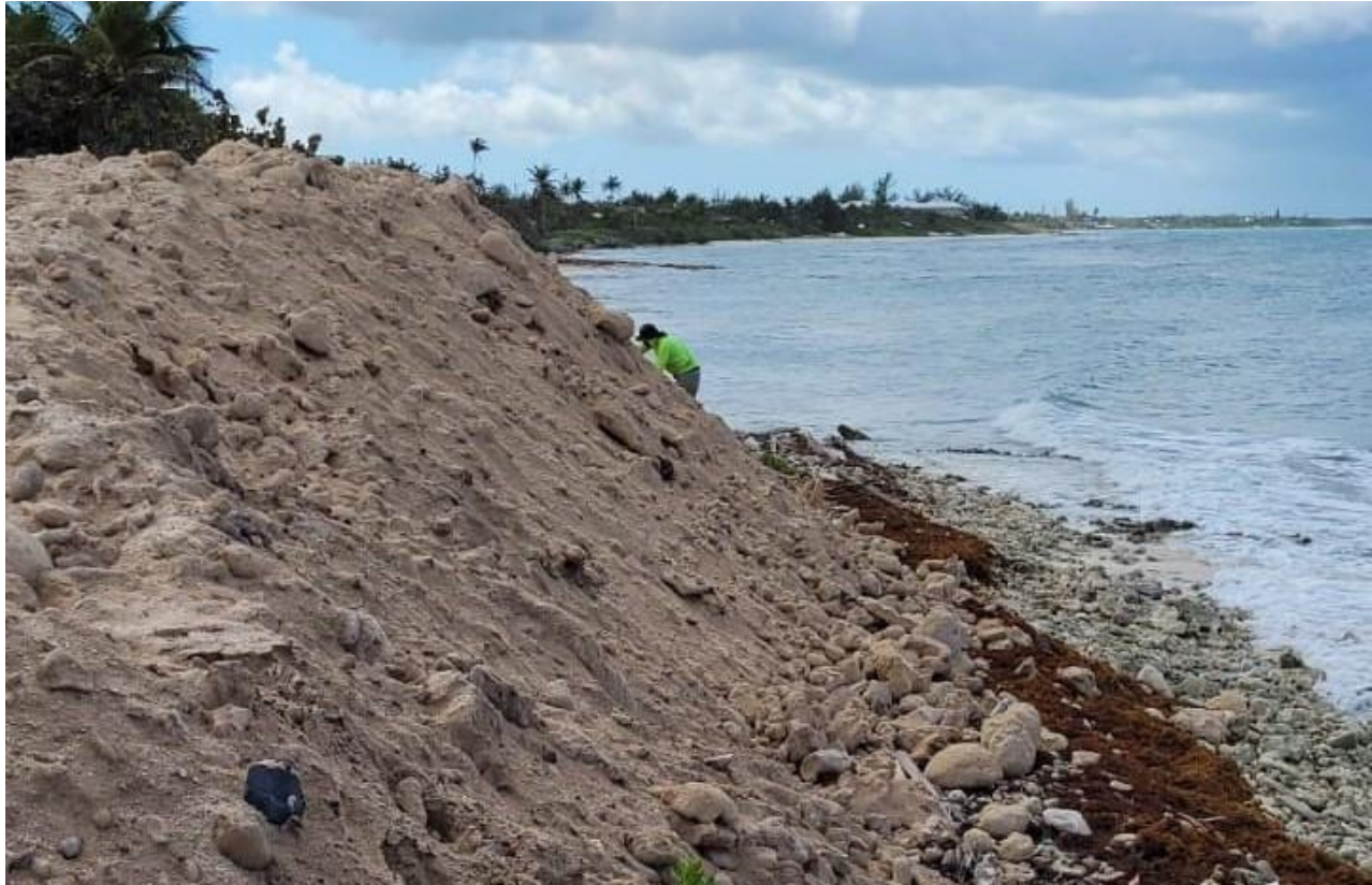
Figure 13. Material stockpiled too close to the water's edge which would or would be likely to enter the marine environment during a storm.
