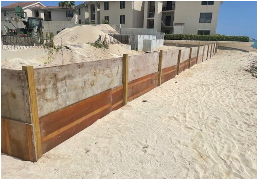
Figure 6. An example of suitable construction fencing to protect turtles (Source: DoE, 2022).
