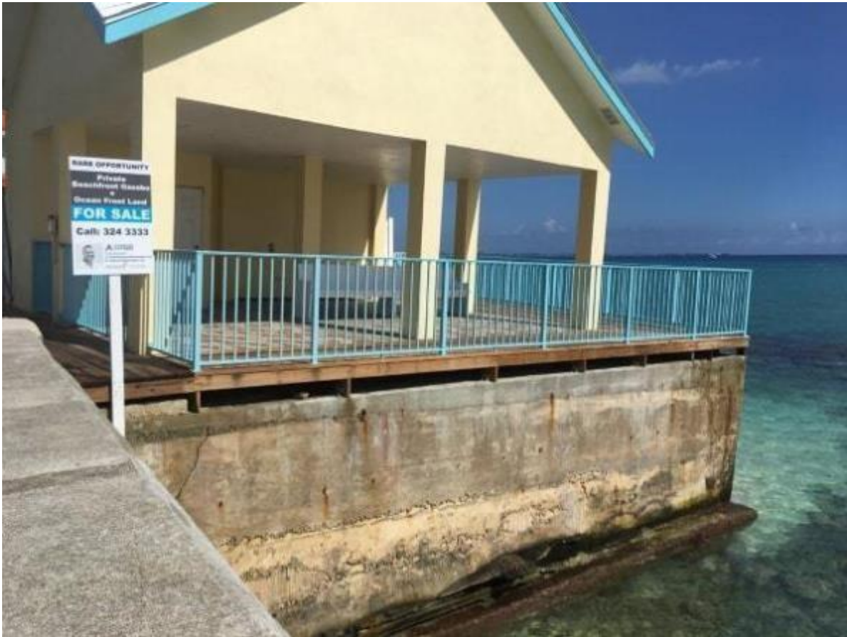
Picture 9: The site in August 2019 (photo from Cayman New Services) shows visible undercutting of the seawall as well as no beach to the south and west of the site.
