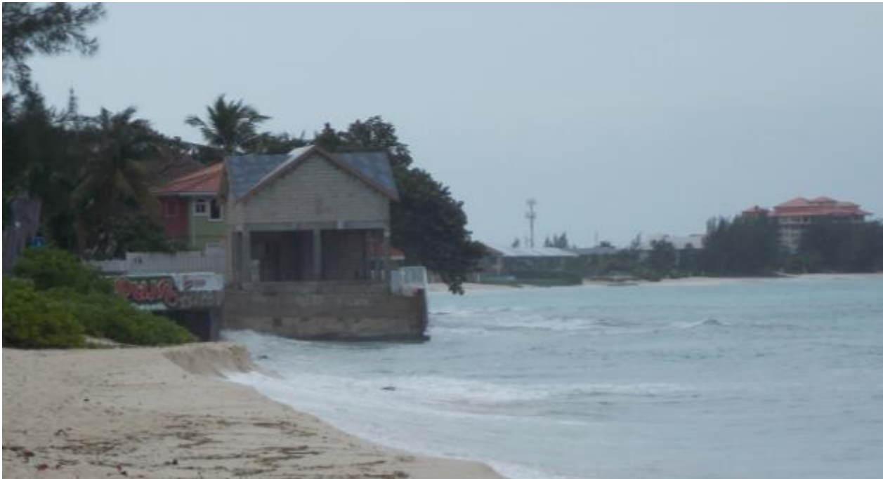
Picture 8: This photo of the site from September 2013 shows that gazebo is under construction and there is no beach on either the west or the north of the site. There are cresting waves along these two sides of the seawall. The seawall appears to be undermined or the footings are exposed.
