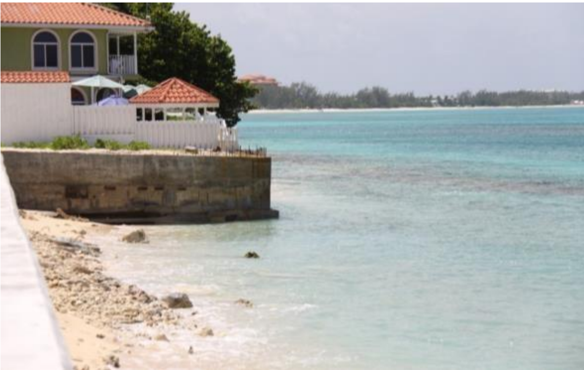
Picture 7: The site in July 2012 shows there was no beach directly in front of the property. The top of the seawall does not appear to be level when compared with previous photos, and the seawall footings are
