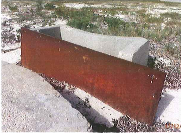
Fig 3: Closed Culvert in South Sound
