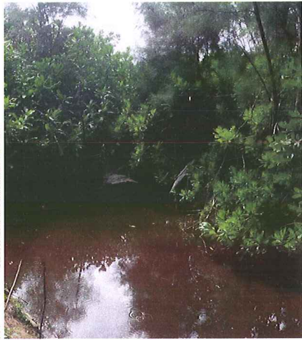
Fig 4: Landward End of South Sound Culvert
