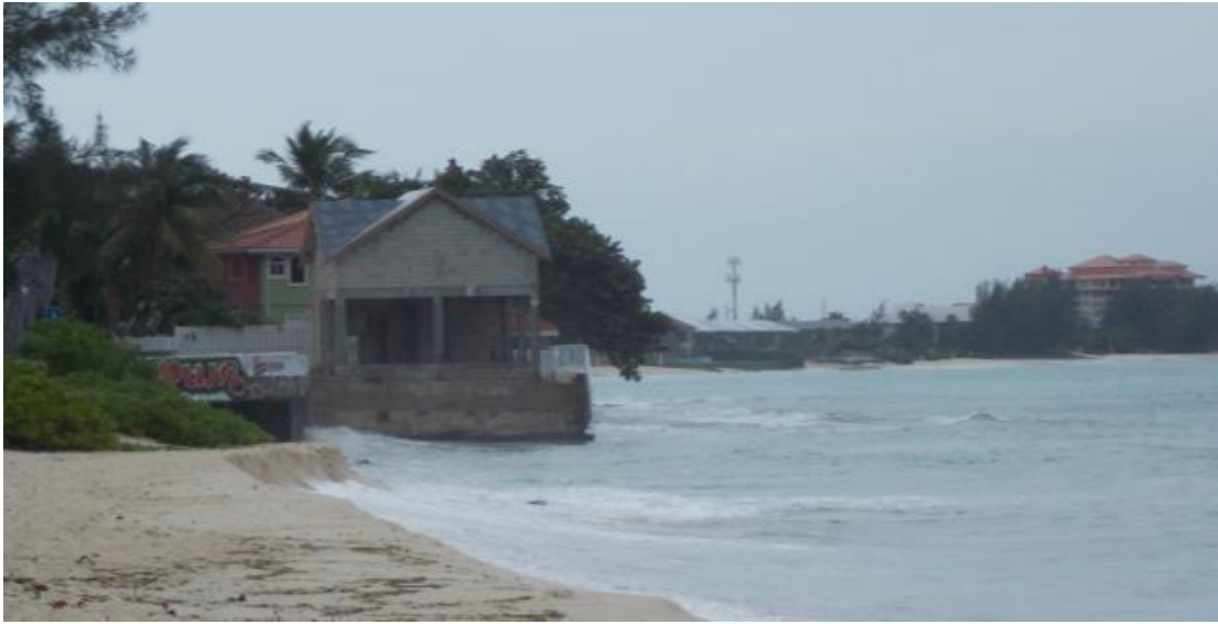
Picture 8: This photo of the site from September 2013 shows that gazebo is under construction and there is no beach on either the west or the north of the site. There are cresting waves along these two sides of the seawall. The seawall appears to be undermined or the footings are exposed.
