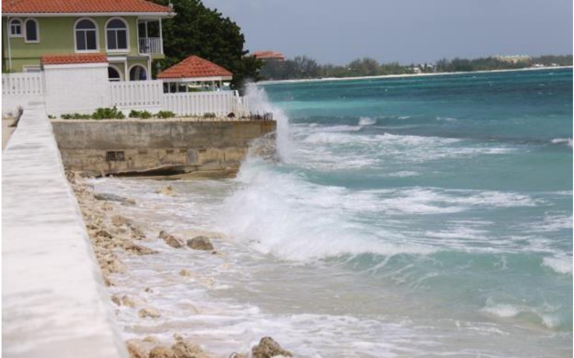
Picture 6: During a period of inclement weather in June 2012, breaking waves can be seen crashing against the seawall and cresting waves can be seen just offshore. The proposed house includes glass railings at the top of the seawall, where the waves can be seen breaking. The living room of the proposed house is just over 5 feet from where the whitewash can be seen.
