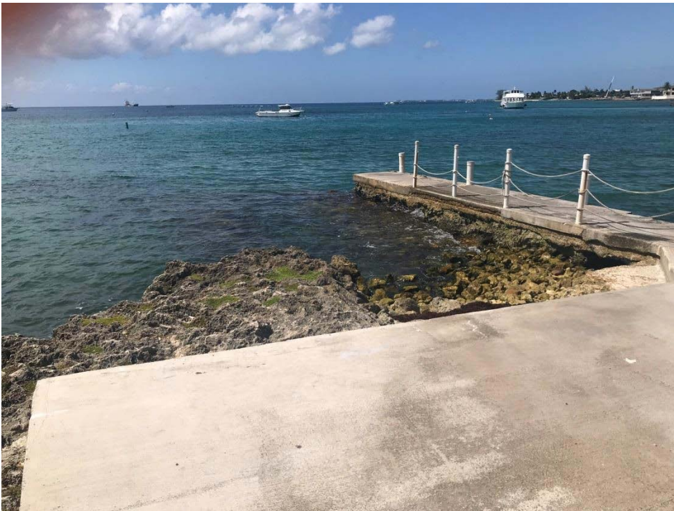
Photographs of After-The-Fact concrete slab and filling of land.
