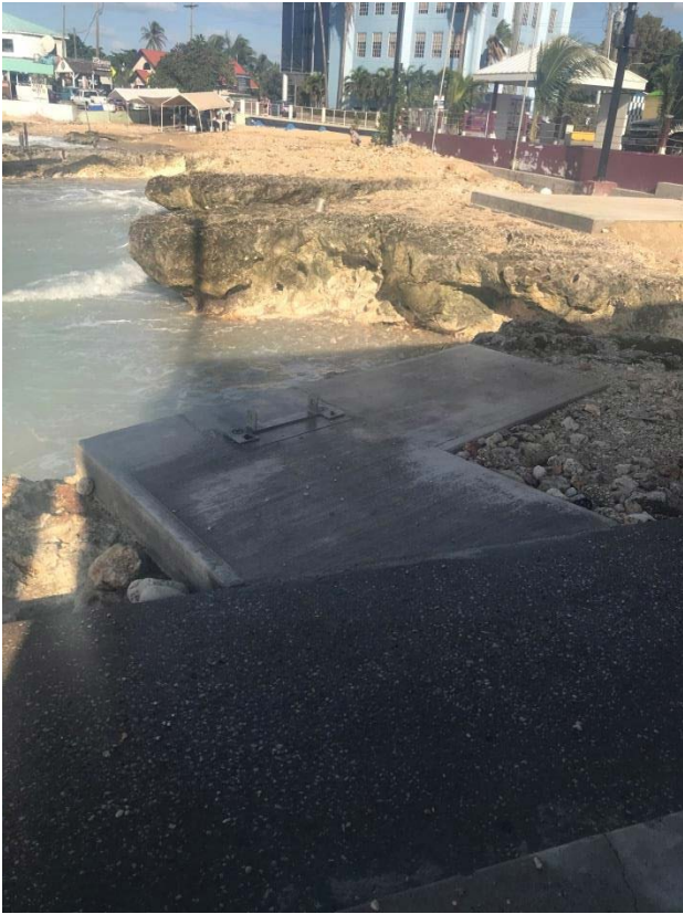
Concrete slab with ladder to enter water.
