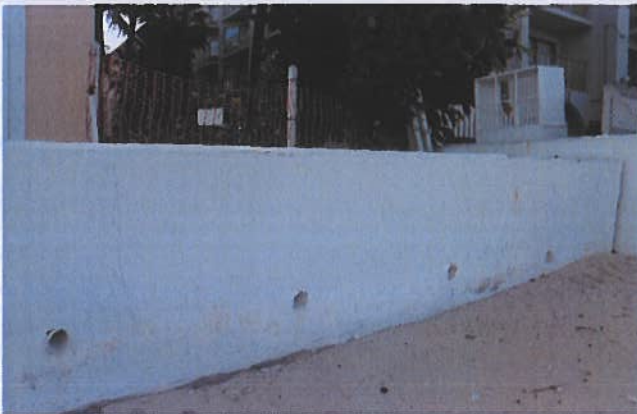
Figure 8: Storm water drain pipes through existing seawall.
