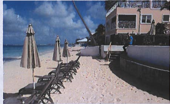
Figure 2: Pool deck seawall at right, upon which person is sitting. Wooden steps from pool deck to the beach, where the pool deck seawall is ‘set back’ from the adjacent seawalls. Damaged seawall in background, left of stairs. Photograph circa Feb 2021.
