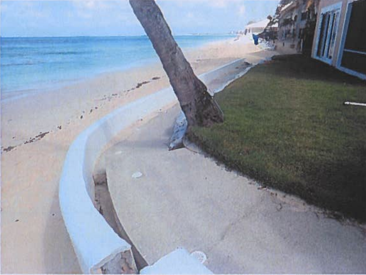
Figure 1 c: Damaged wall looking north (Feb 2021)
