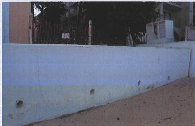
Figure 8: Storm water drain pipes through existing seawall.
