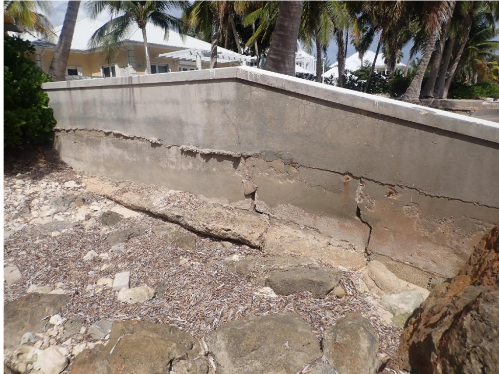
Figure 1. The existing seawall has some cracks and evidence of structural movement.
