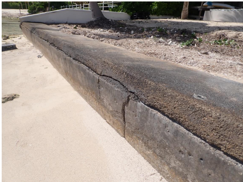
Figure 2. The existing seawall is cracked in places.
