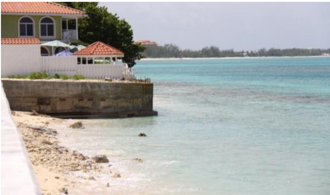
Picture 7: The site in July 2012 shows there was no beach directly in front of the property. The top of the seawall does not appear to be level when compared with previous photos, and the seawall footings are exposed, indicating there may be impacts to the structural integrity of the wall only two years after construction, and prior to the construction of any structures.
