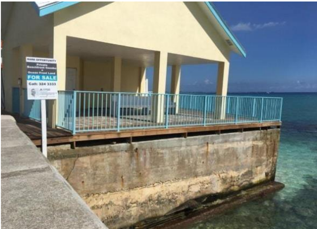
Picture 9: The site in August 2019 (photo from Cayman New Services) shows visible undercutting of the seawall as well as no beach to the south and west of the site.
