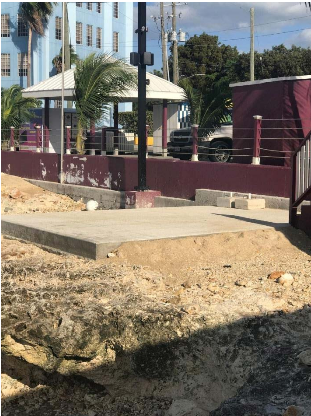
Additional After-The-Fact concrete slab.
