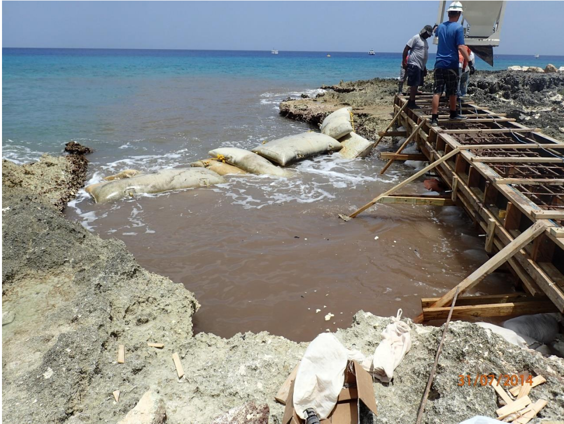
Figure 3: DoE site visit photo from July 2014 showing the sedimentation impacts at a development site on South Church Street using a plywood shuttering method similar to that proposed by the applicant.
