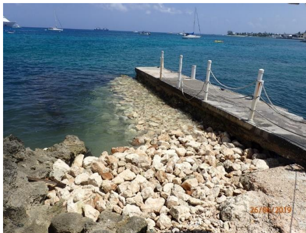
Figure 1: DoE site visit photo showing the illegal filling of the application site in June 2019.
