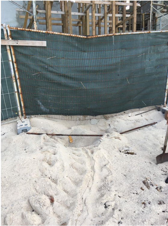
Figures 1-2. Sea turtle tracks showing that the sea turtle has crawled up the beach until it reached a construction site (Source: DoE and Tammy Kelderman, 2021). The fence in Figure 1 is dangerous to sea turtles as it is sharp, rusty and not secure or embedded into the sand.
